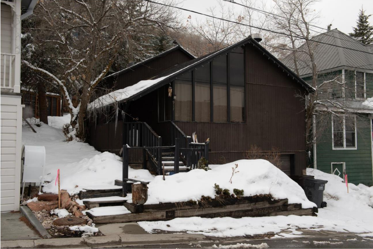
Figure 1: 917 Empire Avenue - Looking Westerly
