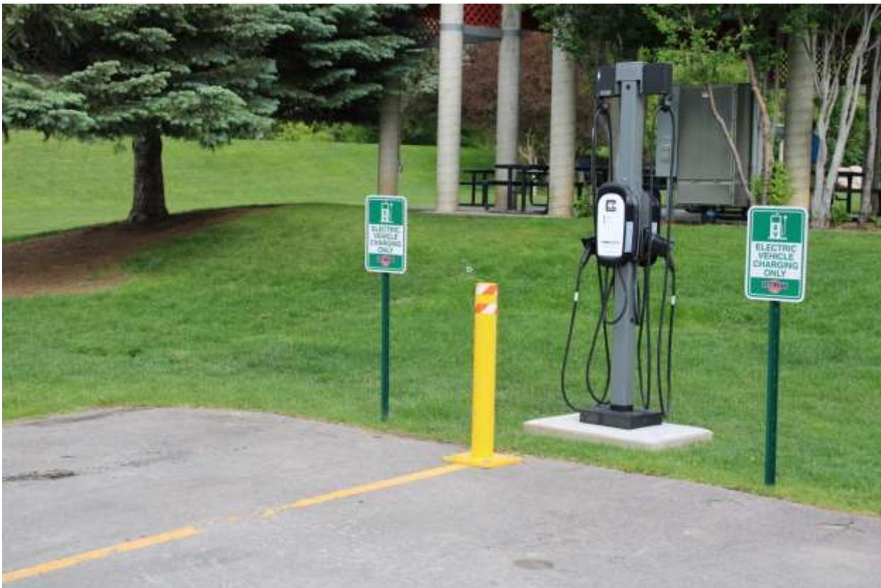
The image above shows the City-installed dual port Level 2 Charging Station at City Park. The City could require the installation of a dual port Level 2 Charging Station at the time of construction for a number of total Parking Spaces.
